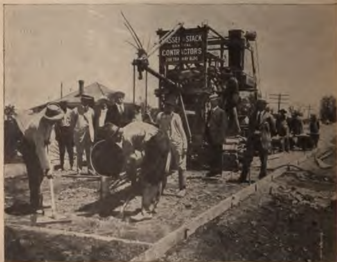
Building a Colorado Road with a Smith-Chicago Mixer.
